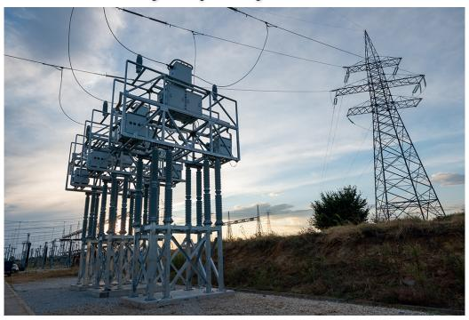
A transformational grid enhancing technology, SmartValve™, has been successfully commissioned in Greece, marking the second deployment of power flow control technology by IPTO. By intelligently controlling the flows of power across the network, this technology can unlock available cross border interconnection capacity between Greece and Bulgaria.
